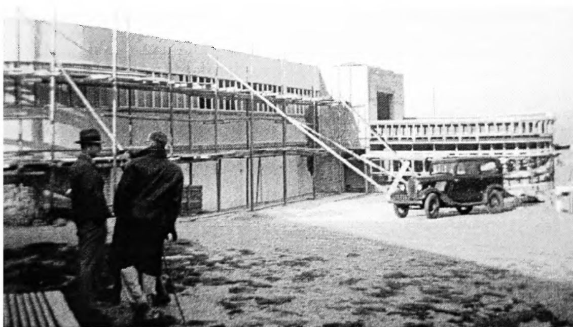
The Clubhouse under construction in 1935 with the wooden scaffolding then in general use.
