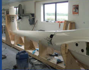
ASK21 in our Jig for fuselage repair
